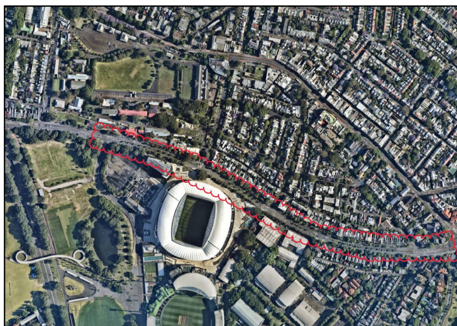
Figure 3.1: Aerial view of the route of the Moore Park Road pop-up cycleway between Lang Road and Driver Avenue
