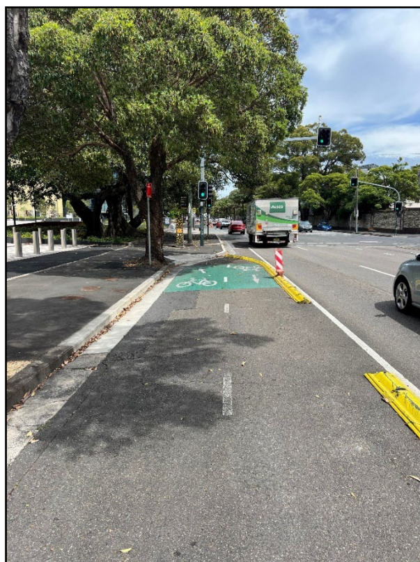
Photograph 3: View looking west opposite Oatley Road, where the cycleway becomes a shared path for a short distance across this intersection.
