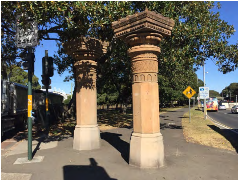
Plate 3.8 Example of the easternmost Moore Park Gateway Piers (view south)
